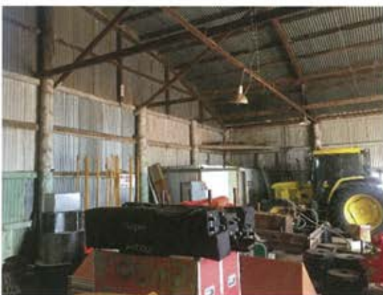
Figure 3.13 Interior of Hangar No. 1 showing framing structure including raw timber log posts. (Source: GML, 2018)
