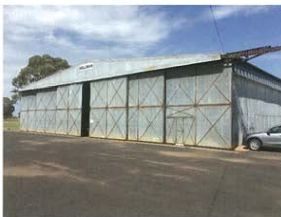
Figure 3.17 Bellman Hangar with outrigger stacking panel doors. (Source: GML 2018)
