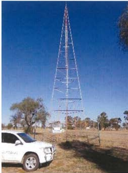
Figure 1: Southern Tower overview. Remnants of layered red and white paint is severely faded and peeling.
