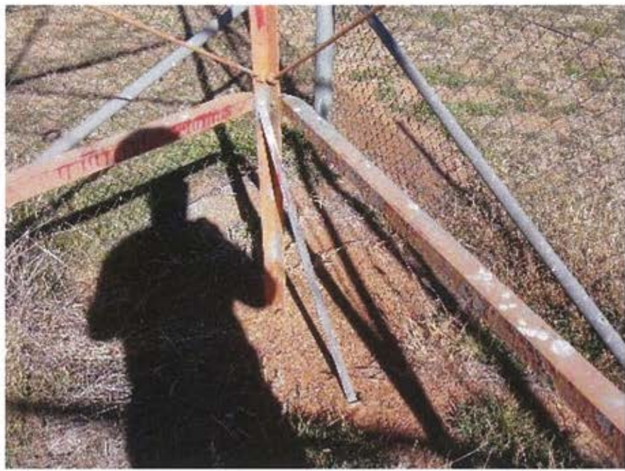
Figure 6 - Typical foundation splice. No evidence of corrosion under the peeling paintwork.
