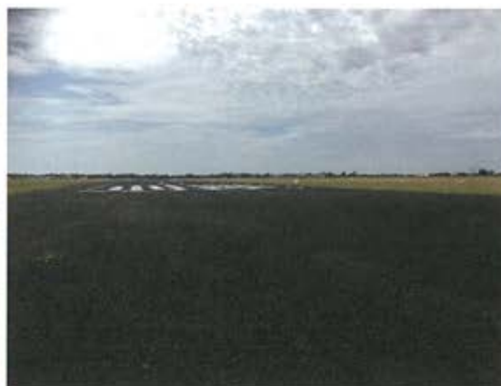
Figure 3.5 Paved runway in the airfield. (Source: GML, 2018)
