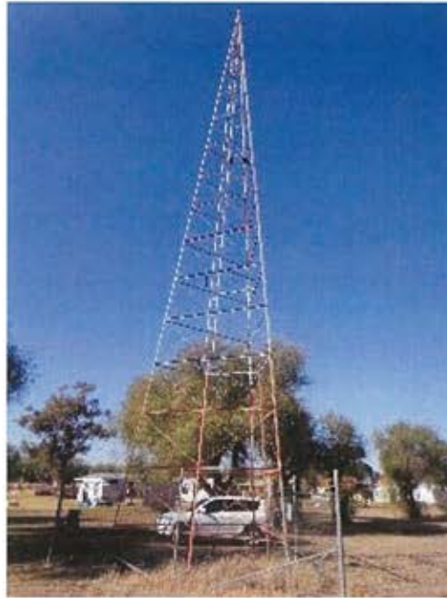
Figure 2: Northern Tower overview. Remnants of layered red and white paint is severely faded and peeling.
