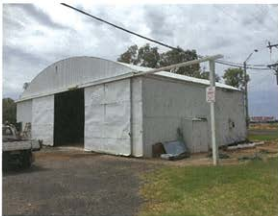
Figure 3.11 Front (ie openable side) of Hangar No. 1 showing outrigger doors. (Source: GML 2018)
