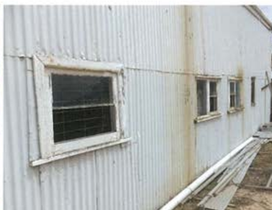
Figure 3.16 Eastern side of Hangar No. 1 showing timber windows in poor condition. (Source: GML, 2018)
