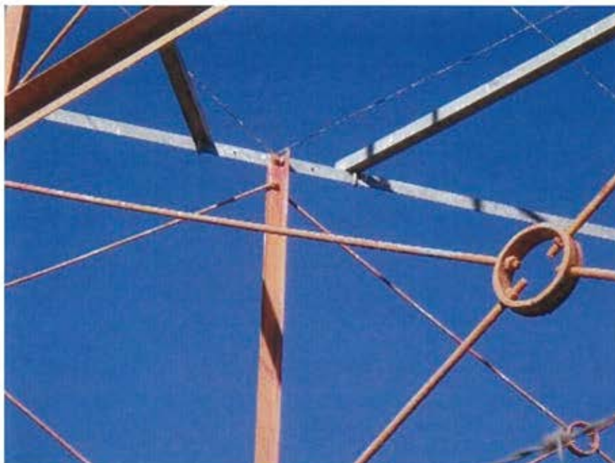
Figure 4: Slight bend in diagonal threaded rod bracing to southern tower.
