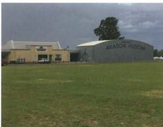
Figure 3.25 Aviation Museum viewed from the former parade ground to the southwest. (Source: GML 2018)
