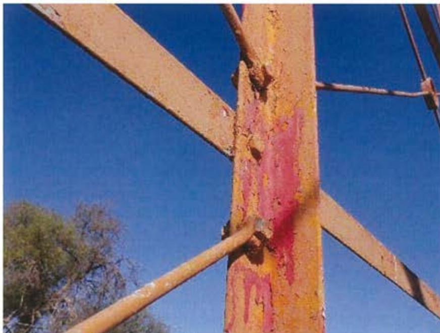
Figure 3: Lower level, threaded rod diagonal brace and centre strut connection. Red paint peeling and faded.
