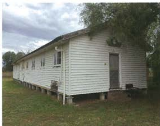
Figure 3.24 Former lesser Qantas building. (Source: GML 2018)
