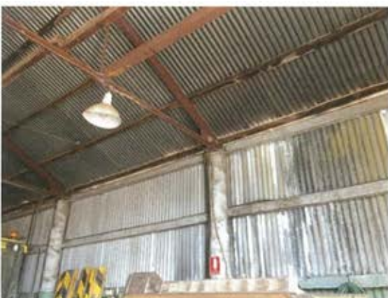
Figure 3.15 Interior of Hangar No.1. (Source: GML, 2018)
