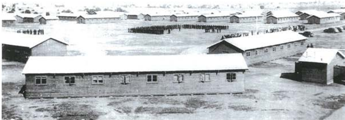
Figure 2.6 View from duty pilot's tower southeast over the base c1940. The headquarters building is in the foreground, the parade ground in the midground with the airmen's and trainees' quarters precinct in the background. (Source: Norma Meadley, Narromine History Room)
