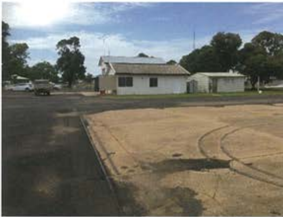
Figure 3.35 Buildings 5, 6 and 7 with the concrete slab of removed Bellman in foreground. (Source: GML, 2018)
