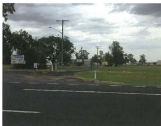
Figure 3.3 Entrance to the aerodrome at Tom Perry Drive on Mitchell Highway. (Source: GML 2018)
