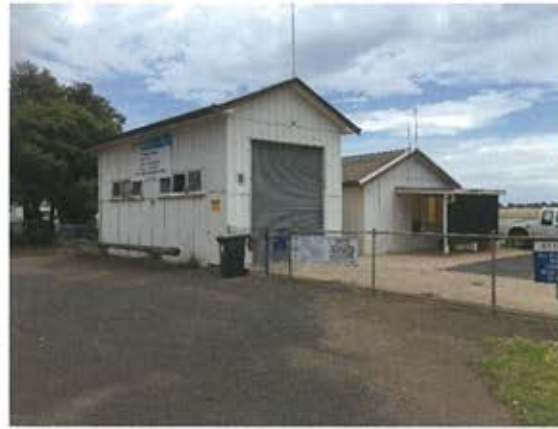
Figure 3.34 Building 5 (left) and Building 6 (right). (Source: GML, 2018)
