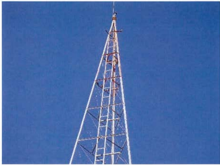
Figure 7 - Top of tower, steel ladder would not comply with current Australian standards.
